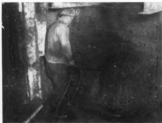
SPILING is driven at working faces for support and safety. Stoper is used here to drill some hard clay.
